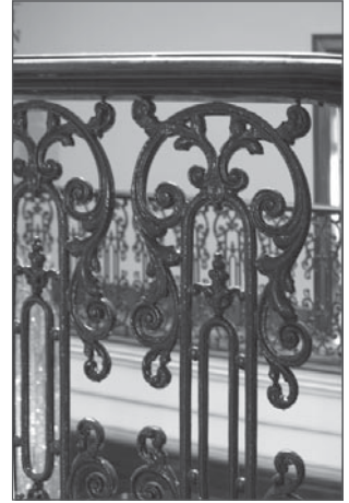
Detail of the upstairs balustrading at Old Government House, September 2009.
