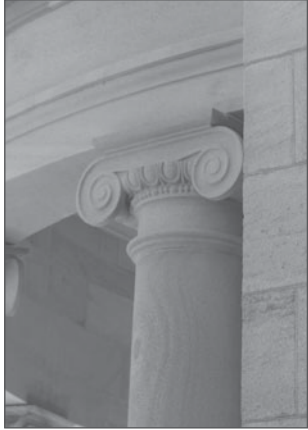
Detail of a column capital at Old Government House, September 2009.
