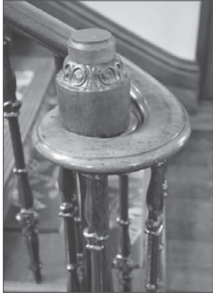
Detail of the balustrading at the bottom of the main staircase in Old Government House.
