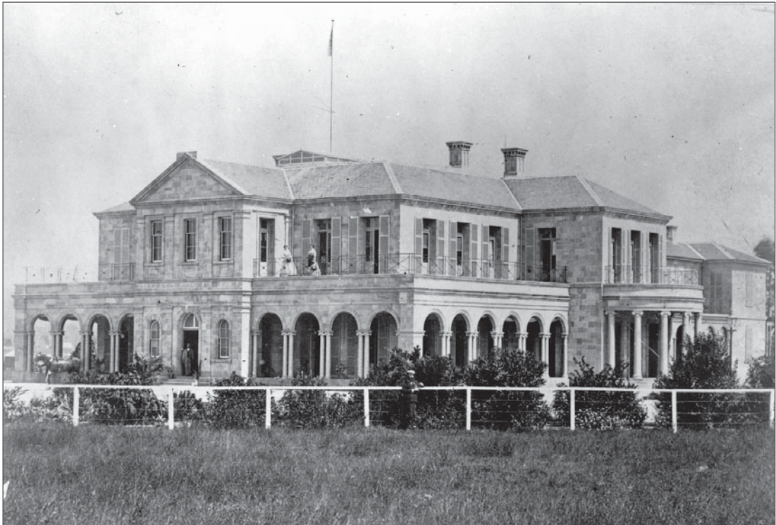
View of Old Government House prior to the upstairs verandahs being covered. c 1863. State Library of Queensland Neg No. 3801
